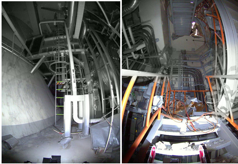
Fig. 1 High-resolution photos captured in the reactor building of unit 3. The left shows the piping of the core spray system and the right shows the rubble blocking the staircase to the third floor.
