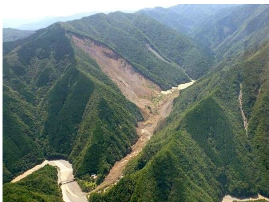
Fig. 1: Akatani natural dam (Gozyo City Nara Pref, ©Ministry of Land, Infrastructure, Transport and Tourism : MLIT)
