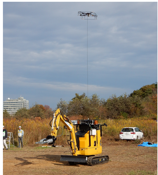
Fig.1: Field test of the developed Helipad
